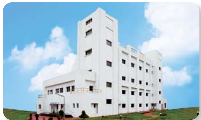
API Facility, Roha
